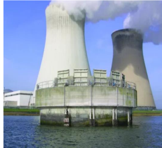
Figure 7.2: Doel power station with (left) estuarine intake and (right) AFD units
