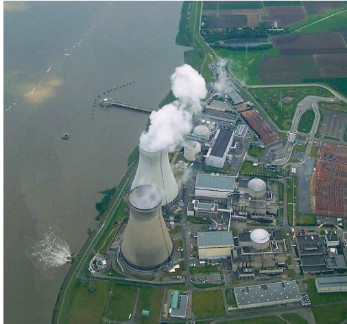
Figure 7.2: Doel power station with (left) estuarine intake and (right) AFD units
